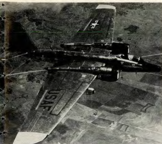
RB-57F, high flying reconnaissance aircraft samples upper air for nuclear debris.
